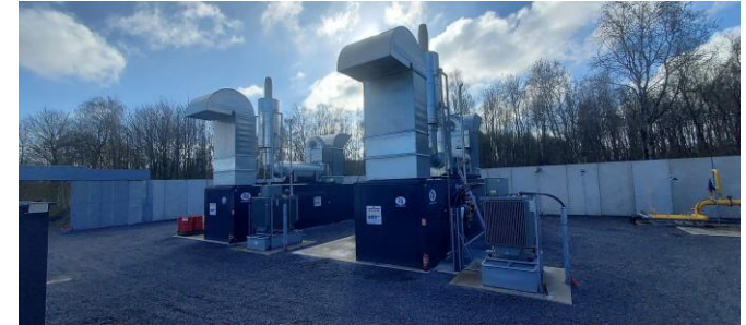
Installation completed for the two units at Angres in northern France
