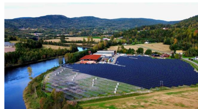
Installed solar photovoltaic panels in Engene, Norway
