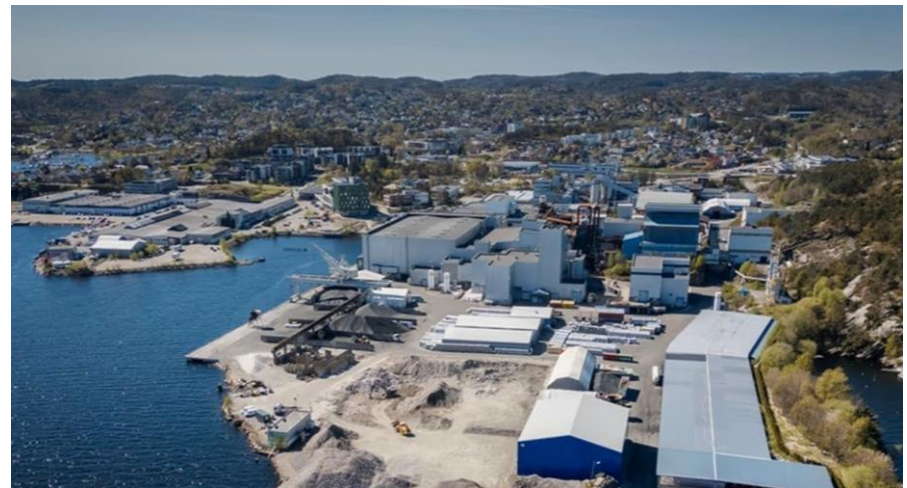
Planned H 2 plant at Agder
