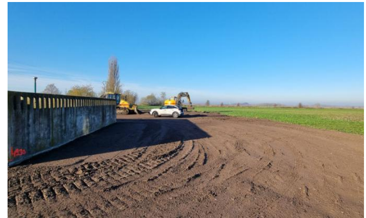
Beginning of the construction in Rouvignies site
