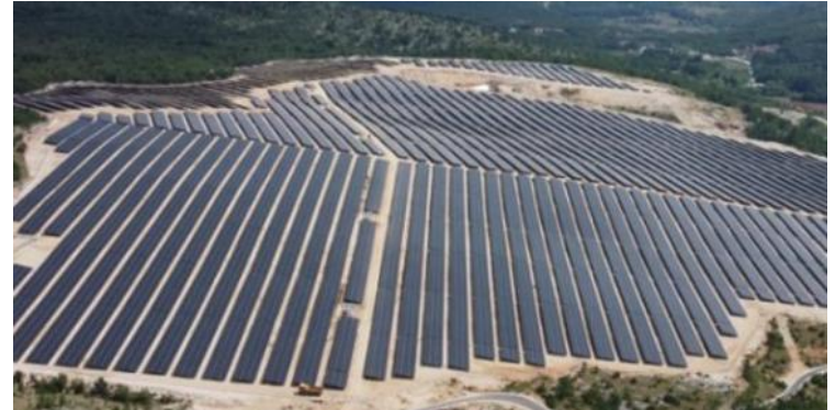
Installed solar photovoltaic panels in Petjnik, Bosnia
